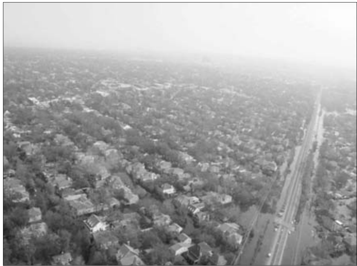
Devastated areas of New Orleans as seen from the Kaspers' helicopter.
