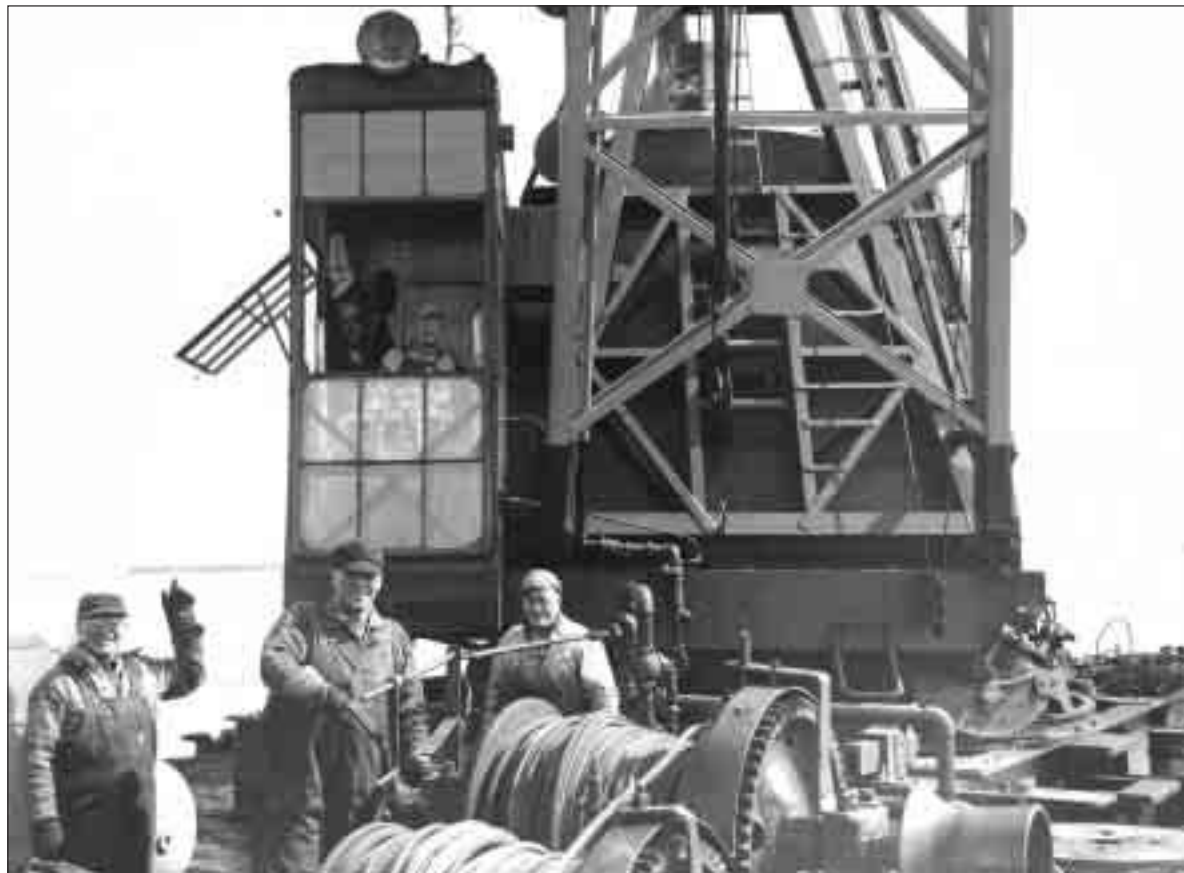
The late George Saunders (far left) stands with his derrick crew during the construction of the Mackinac Bridge, which opened in November 1957. Derrick operators were responsible for lifting steel beams and personnel more than 100 feet in the air, manipulating 14 levers to operate the derrick's 160-foot boom. (Photograph courtesy of Richard Saunders)
