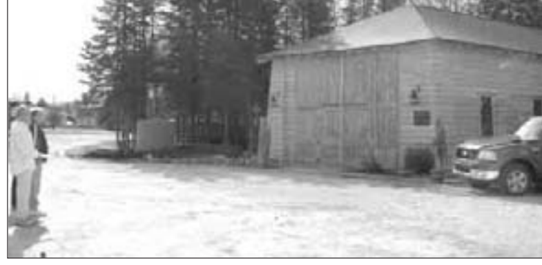
Michael Miller and Lyle Nordquist of the Les Cheneaux Historical Association survey the extensive renovations, including new pine siding, that brighten the outside of the Les Cheneaux Maritime Museum in Cedarville. The front door of the historic boathouse was corn blasted to reveal the bright, clean wood underneath its weathered exterior.
