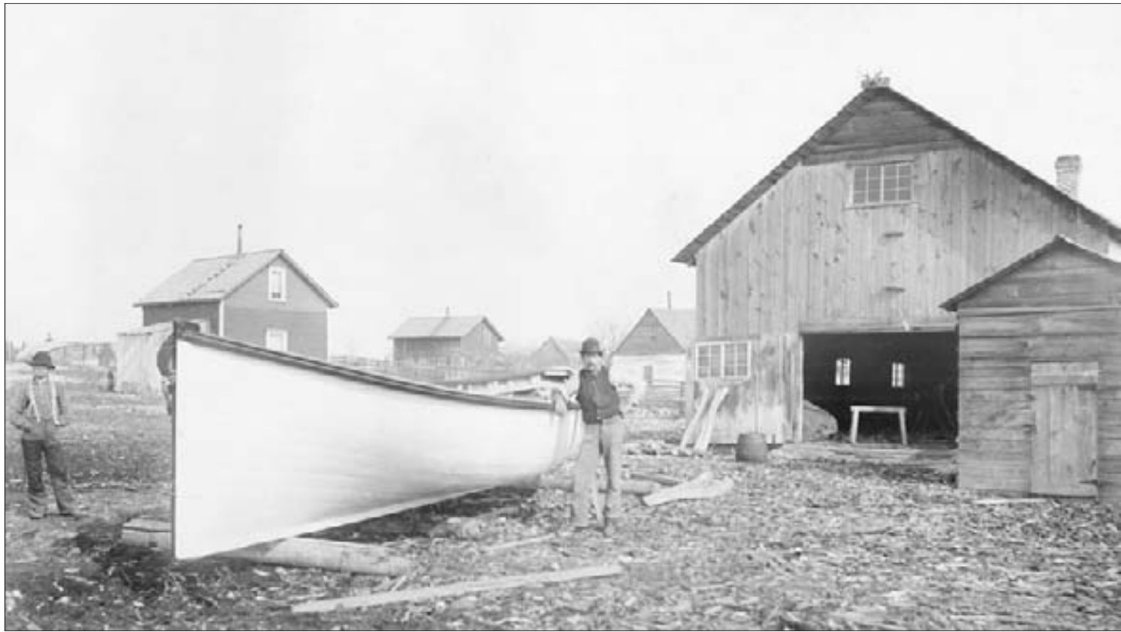
Standing next to a newly built Mackinaw boat are Ignace Cheginer (middle), and, on the far left, Jimmy Pond, at Mr. Cheginer's shop. Mackinaw boats are a strong, flat-bottomed boat used by fur traders and had evolved into a type of sail boat for open water. Just behind the barn is the Grondin family log home, which would be on what is now called Grondin Street in St. Ignace, near the Mackinac County airport. According to the writing on the back of the photograph, it was torn down in the 1960s. At the far left is the home of Thomas Cheginer, which was destroyed by fire in 1941. The building in the middle is unidentified. The lumber in the barn and shed, according to an inscription on the back, was used to build the Mosier home, near the present day Mackinac County Road Commission building. The photograph was taken in the 1880s. (Photograph courtesy of Paul Grondin)
