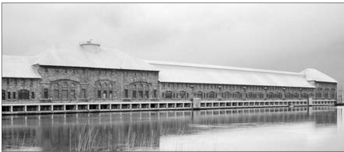
Edison Sault's hydro generating plant on the St. Marys River in Sault Ste. Marie began generating power in 1902. In 2007, the plant is estimated to produce 36 percent of the company's electric power.
