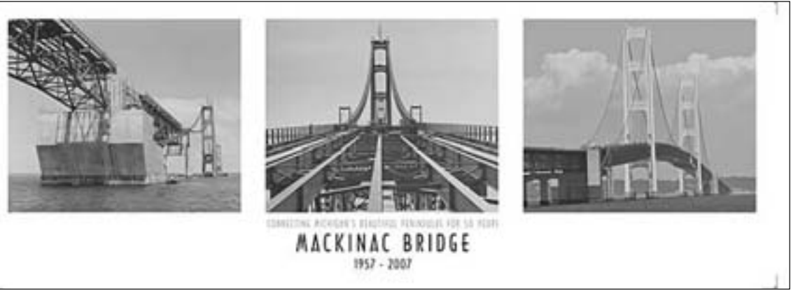
This is one of four posters available from the Michigan Department of Transportation that marks the 50th anniversary of the Mackinac Bridge. (Photograph courtesy of the Michigan Department of Transportation)
