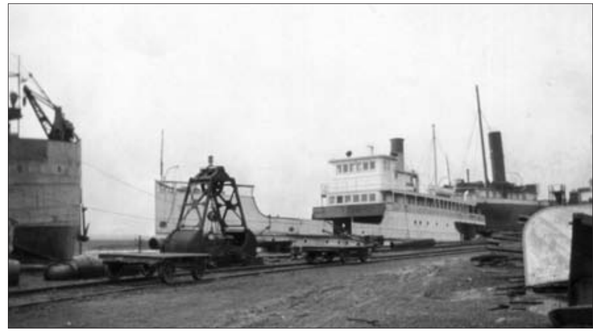
After a harrowing early winter voyage up the lakes to a Detroit shipyard, the Colonel Card and Colonel Pond were cut in two and a 50-foot extension was added to each ship's bow. They emerged as the Michigan State Ferries Mackinaw City and Sainte Ignace and entered service at the start of the 1924 season. (Snapshot from author's collection. Photographer unknown.)
