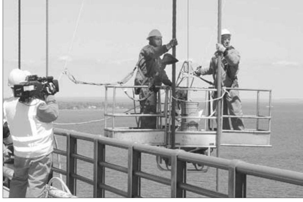
Secured to the Mackinac Bridge and the spider climber with multiple safety lines, bridge steeple jack Fred Spinella (left) and Mike Rowe prepare for painting suspension cables Friday, May 25. Their work is captured by a Discovery Channel cameraman standing on the bridge deck and a camera crew in a nearby spider climber. (Photograph by Dan Johnson, MBA)
