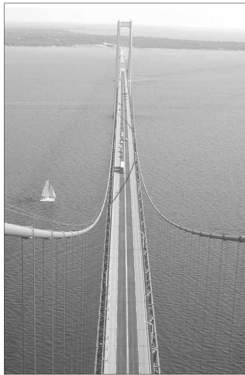
Michigan's superstructure, the Mackinac Bridge, celebrating its 50th anniversary, was named Michigan's best landmark by The Detroit News ' "Michigan's Best 2007" readership poll. The view is from the top of the south tower facing St. Ignace.
