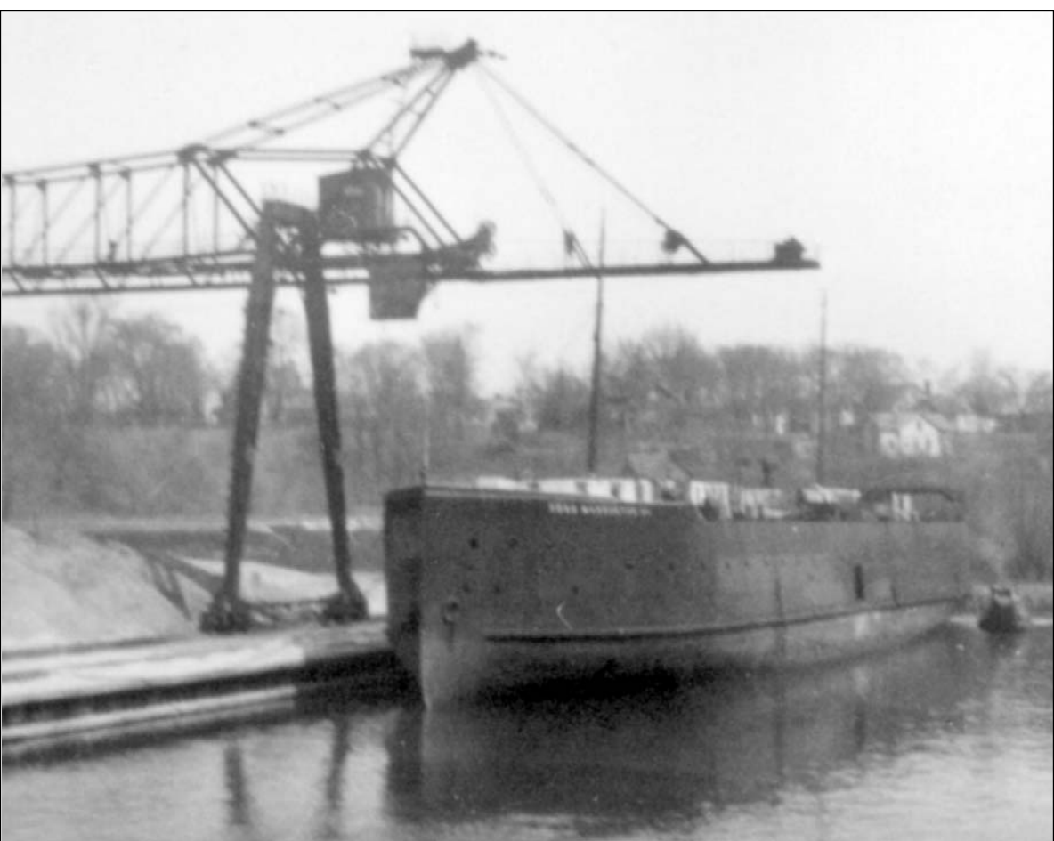
Work began to convert the ferry on March 23 by ripping the rails off her cardeck. Over the next few weeks, cranes removed her pilot house and superstructure, and her dilapidated boilers were removed, to be replaced by a better set, taken out of the Pere Marquette 15 . (Michigan State Archives)
