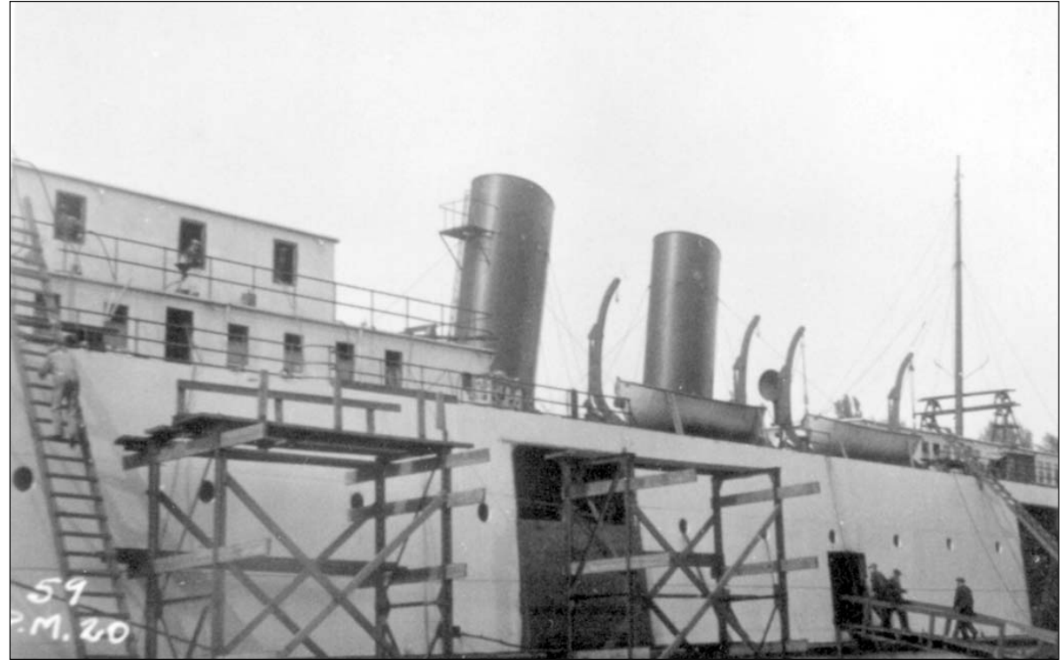
No one brought a set of plans for the existing ferries at the Straits, so engineers had to have someone quickly measure the side loading openings on the City of Cheboygan so the new ferry could be built to match. The openings were quickly cut into her sides. New funnels were fabricated and installed along with a whole new superstructure. (Michigan State Archives.)
