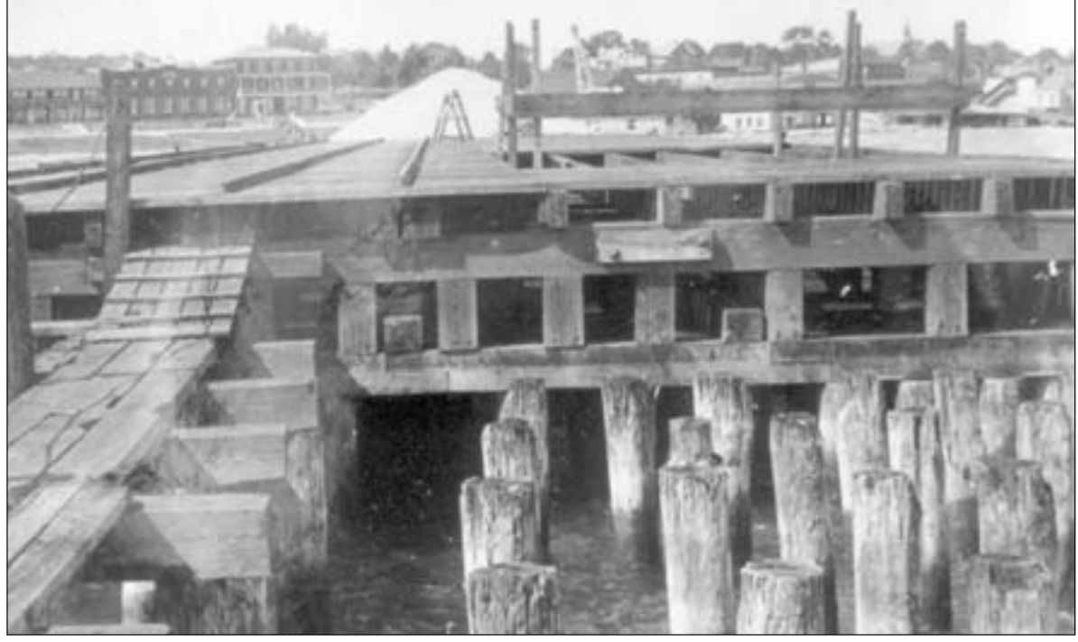
Workers cut beams and huge planks to surface the new end-loading slip, formerly the ferries' coal dock in St. Ignace. This is the site that would come to be known as "Dock 2." In the background, just to the left of the white gravel pile, is the Nicolet Hotel, a popular watering hole for ferry workers and much of the city, as it had one of the few bars licensed to reopen at the end of Prohibition.
