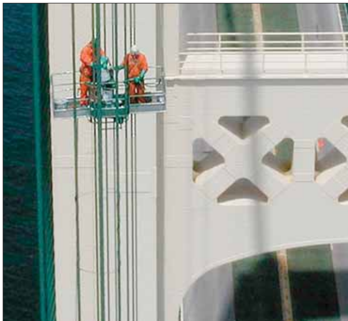
An unidentified maintenance worker (above) performs early paint work on the bridge while standing in a barrel. Crews today use a spider climber (below) and are secured with multiple safety lines. The modern painting process remains similar, as a worker runs his paint-soaked gloves down the bridge cables to add a fresh coating of paint. (Photograph courtesy of Mackinac Bridge Authority)
