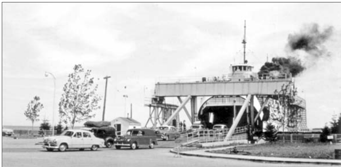
Here is the City of Cheboygan discharging autos in St. Ignace. With two railroad ferries, four auto ferries, and several of the Mackinac Island passenger ferries all powered by coal-fired steam boilers, residents had to keep close track of wind direction before hanging laundry out to dry. Of all the large ferries at the Straits, only the Vacationland was diesel-powered, although by the end of the decade, Arnold Transit would also be switching to diesel boats. (Author's collection)
