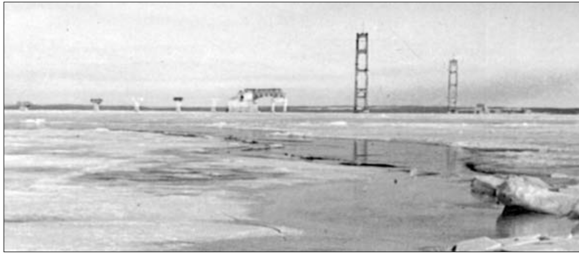
Just before marine operations shut down for the winter of 1955-56, steelworkers installed the first two truss spans that would form the roadway of the Mackinac Bridge. The view of the structure's progress served to remind ferry crewmembers that their jobs would soon be ending, and it stimulated them to seek better compensation and benefits from the Civil Service Commission, which handled labor issues for the Michigan State Highway Department. (Detail of Hiawatha Post Card, author's collection)
