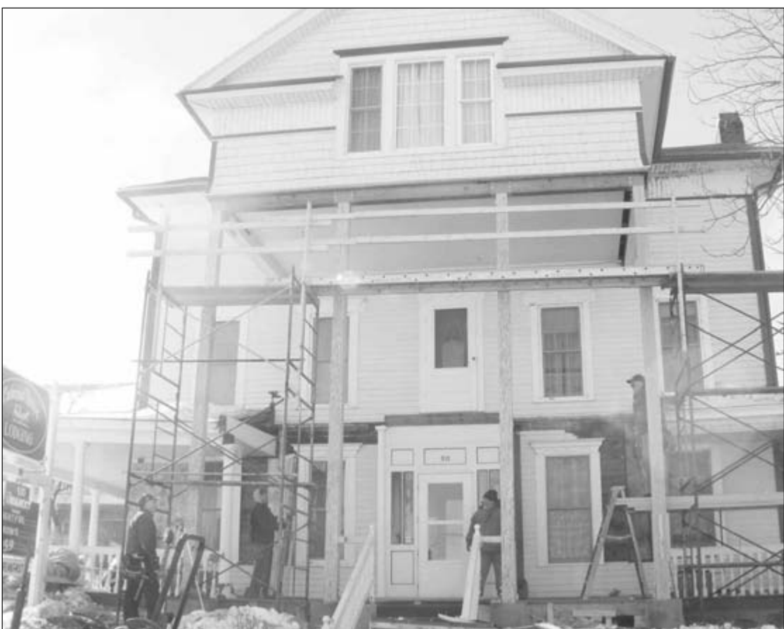
Top: The four front porch columns on the Colonial House Inn in St. Ignace are being replaced by Marshall Builders, owing to wood rot. The inn, built in the mid-1800s, is expected to be open by March, said owner Chris Green. She is also redecorating the inn's former gift shop, on the north side of the building, as a gathering room for groups. Ms. Green said the room should be ready by summer. The three-story building includes seven Victorian rooms. A 10-room motel is connected on the south side.
