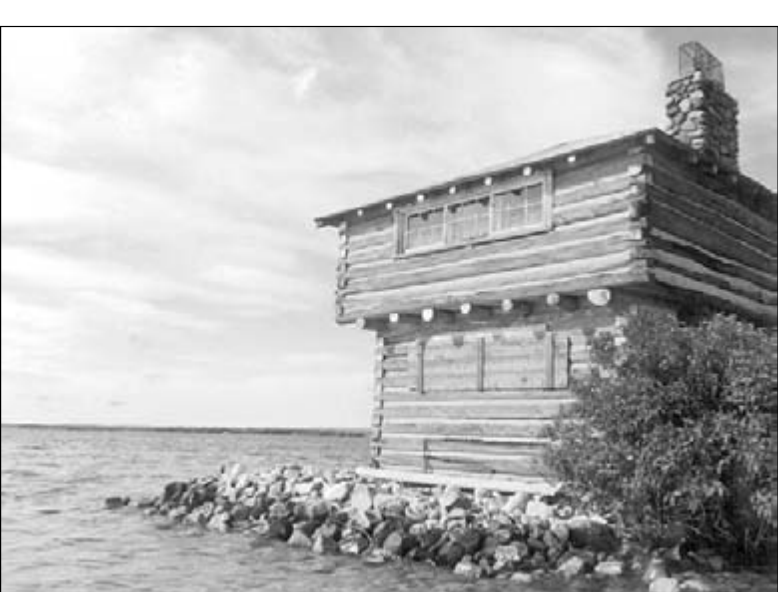
The 98-year-old Long Island Blockhouse at the West Entrance of Hessel will be demolished and rebuilt in the same style of log construction. The stone chimney will not be rebuilt, but the distinctive profile of the building will remain as it has for nearly a century. (Photograph by Joe Eger)
