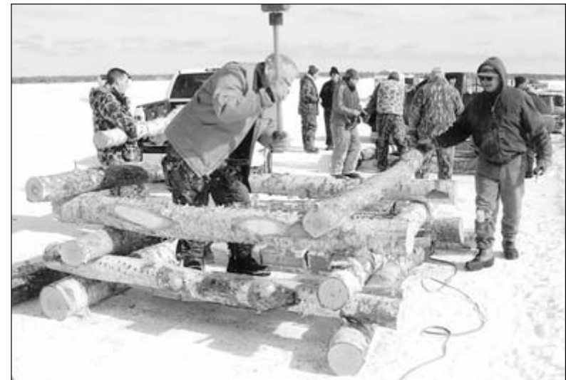
Keith Doepker hammers a spike into a fish crib on Brevort Lake Saturday, February 28, while Ray Lowetz holds the log in place. (Photograph by Louis Colegrove)
