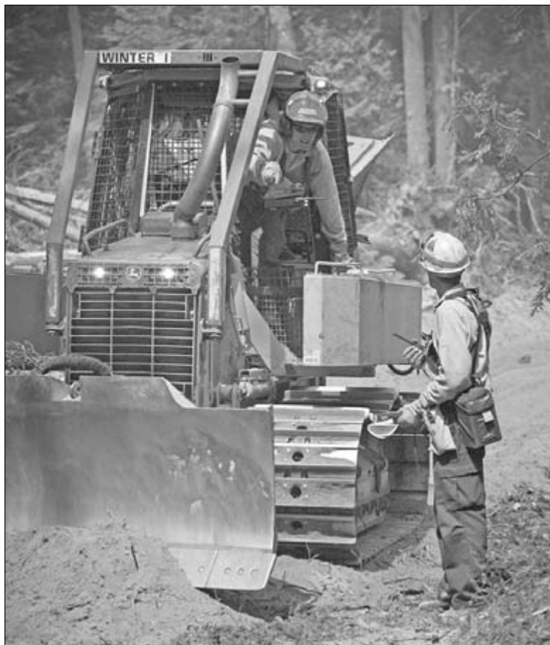
Heavy equipment, such as this tractor/plow that is used to build a fire line, is the backbone of fire suppression efforts in Michigan.
