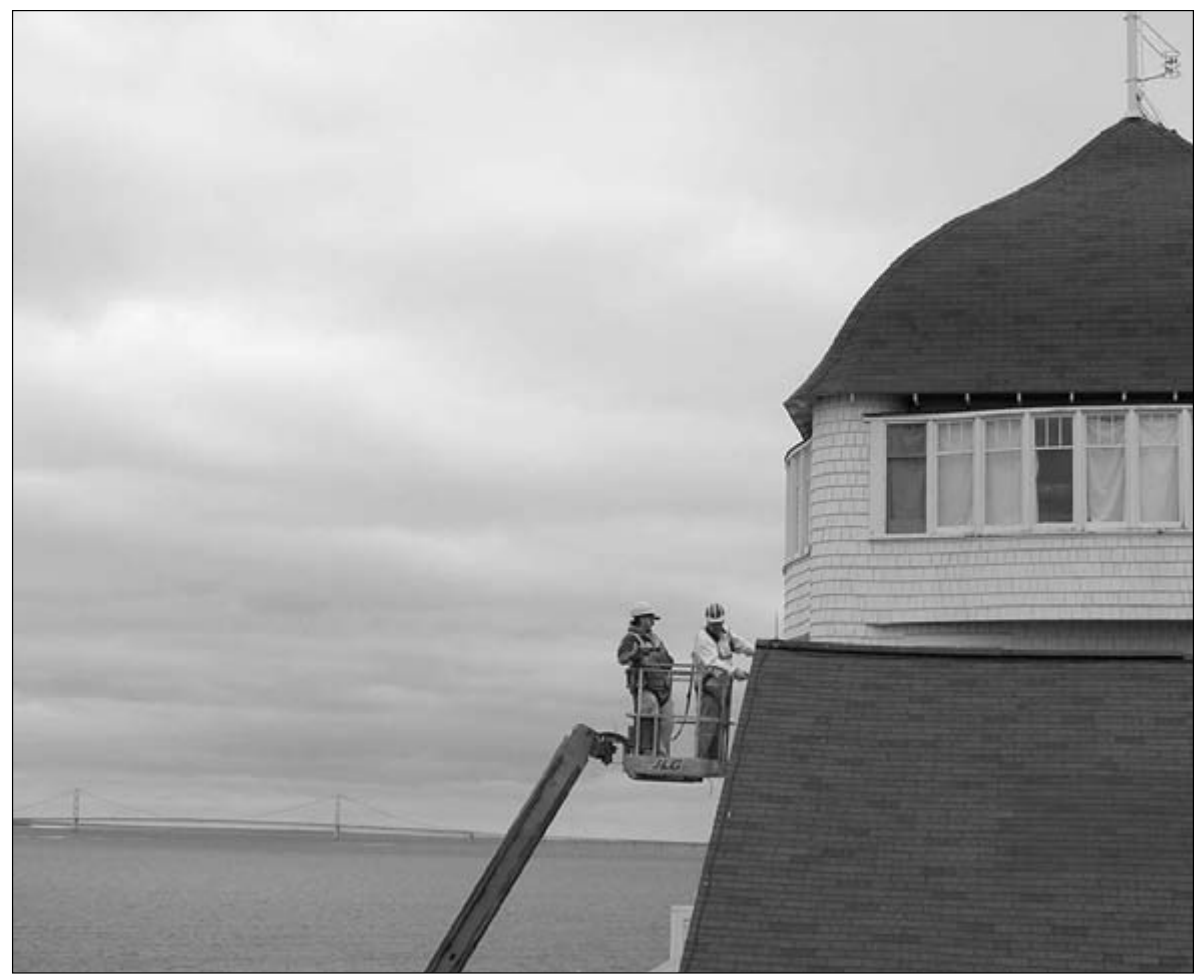
Preparing for the season...With the Straits of Mackinac and the Mackinac Bridge as a background, painters Kirk Smith (left) and Jason St. Onge, standing on a lift 80 feet above the ground, scrape paint near Grand Hotel's cupola on Mackinac Island Tuesday, April 7. Grand Hotel will open for a Rotary conference Friday, April 24. The visitors will get a peek at work needed each spring to open the hotel. Painters will use more than 200 gallons of paint for the hotel's front porch, balconies, ceilings, and flagpoles.
