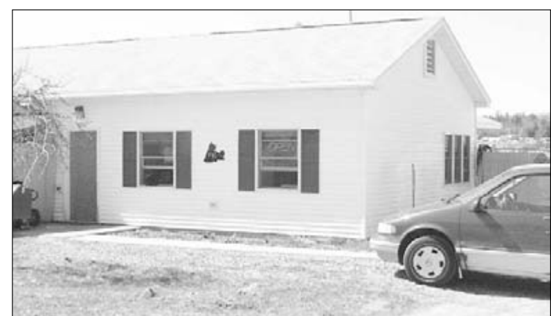
Construction will begin in May on an addition to the county's animal shelter on Cheeseman Road in St. Ignace. The new playroom for cats will be attached to the side of the building near where this vehicle is parked.
