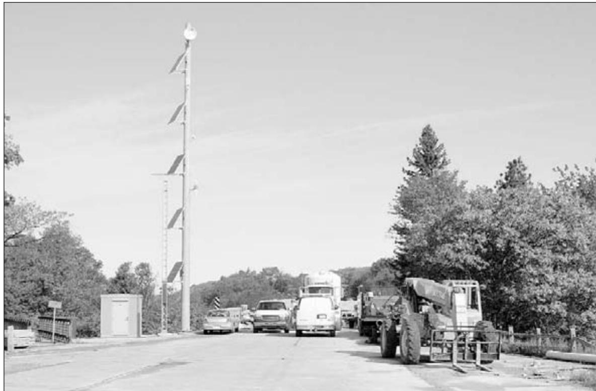
Two towers at the east entrance to the Cut River Bridge along US-2 will report real time weather conditions and bridge data beginning this fall. The first pole, an aluminum fold-down tower, is 30 feet tall. The second, much larger pole supports five solar panels used to operate the system. Radio communications is at the top. The small building contains computer equipment. Vehicles now block the entrance to the bridge, Thursday, June 11, as crews work on renovating the span.
